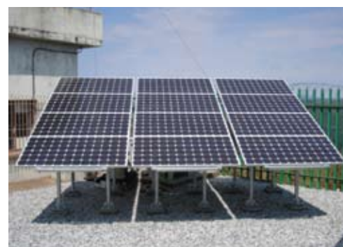
Solar panels powering 'no frills' base stations in South Africa
