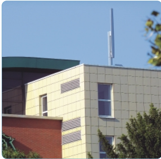
Almost 80% of Vodafone Netherlands installations are on rooftops.
