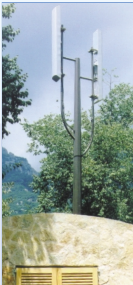
A Vodafone Spain base station sited close to Alfabi Gardens near Soller (Mallorca). The antennas and mast have been designed to simulate the outline of a cactus with the cabin enclosed in a stone-clad structure.
